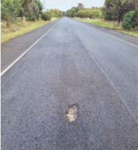
This hole appeared on the road to Rendelsham within days of roadworks being completed there. The hole has since been repaired. Picture: SUPPLIED
